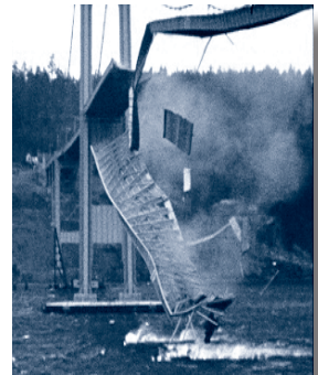
Collapse of the Tacoma
